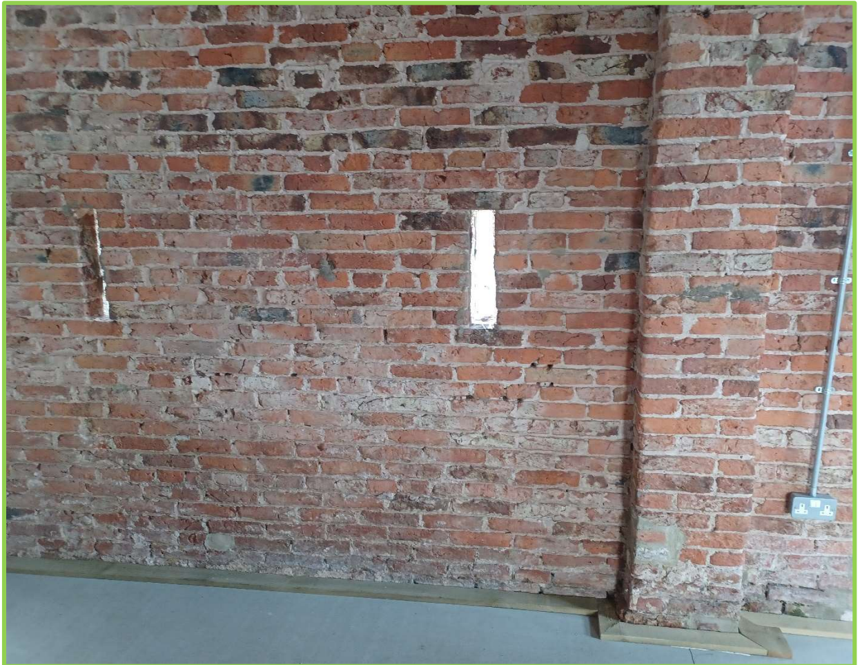
Drawing 15: Glazing Filled Gaps, Eastern Façade of Rustic Barn
