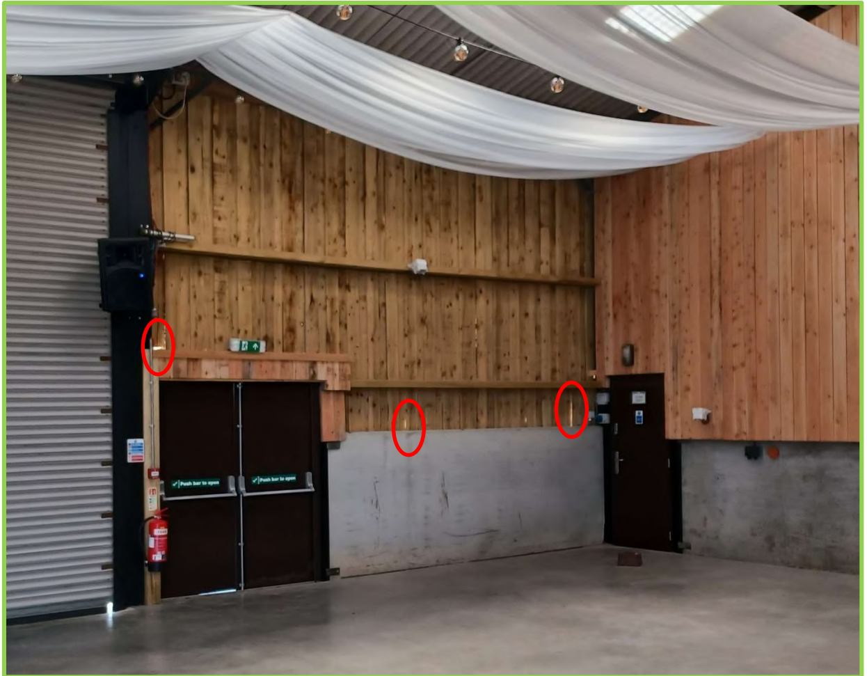
Drawing 8: Gaps between overlapping Yorkshire boards
